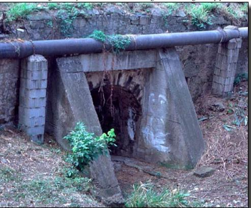
P3.2.6.1 The Bridge as seen from the north side showing the blemishing water pipe.
