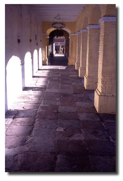
*P. 3.3.3* Pavement build with Oland stone. The Christiansted arcade exists because of an urban plan that allows building an overhang to the first floor, therefore hanging over the pavement.
