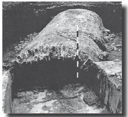
*P* 3.2.14.2 Drain made of conks. Under maintenance the old drains have been demolished by mistake and new drains were established.
