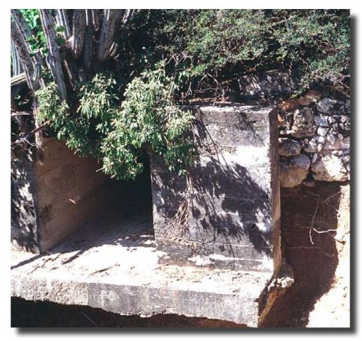
*P* 3.3.4 Old Bridge at Fareham Estate. The concrete extension was built in later to prevent erosion.
